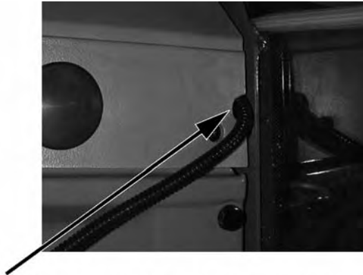
FRONT STEERING CONSOLE - CUT HOLE TO ACCESS POWER SOURCE FOR SWITCH BOX
