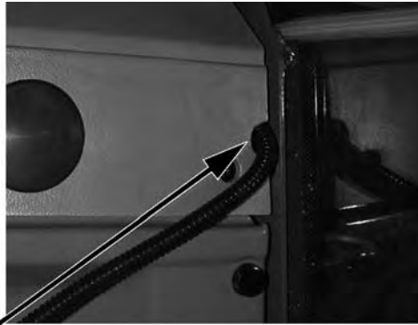
FRONT STEERING CONSOLE - CUT HOLE TO ACCESS POWER SOURCE FOR SWITCH BOX
